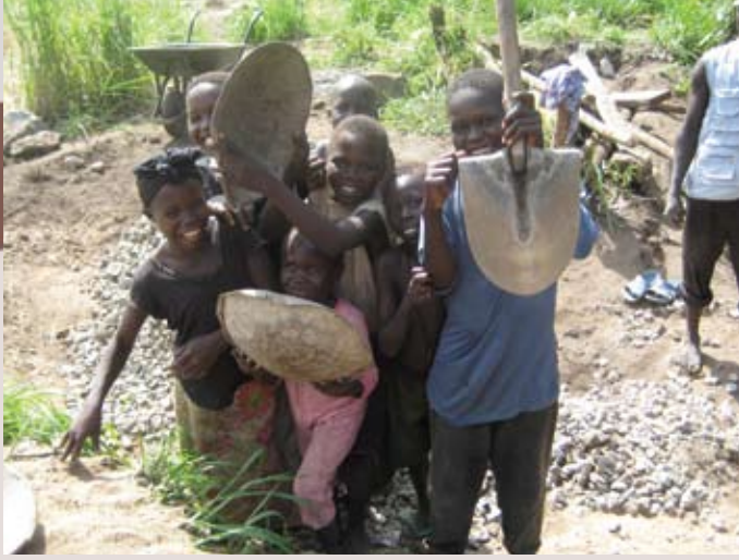
The children who were helping to build the bridge
